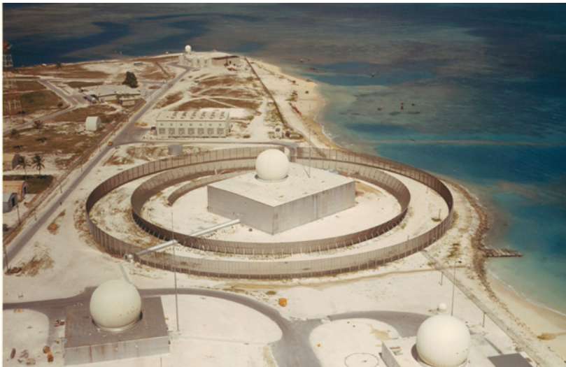
Left: A view of the discriminating radar (inside the clutter fence) and two of the target tracking radars (outside the clutter fence). 7 Right: The discriminating radar antenna beam characteristics, which demonstrates how the cassegrain focus adjusted the beam focus. 8
